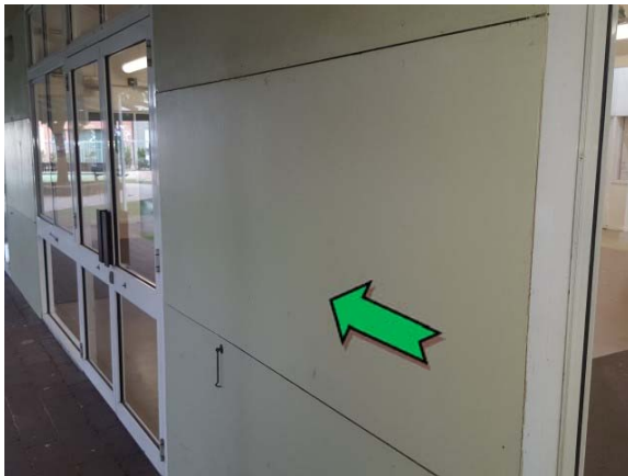
Photo 3. Exterior, throughout, walls – non asbestos-containing fibre cement sheeting.
