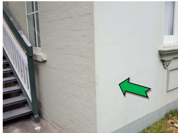
Photo 4. Exterior, throughout, walls – non asbestos-containing textured coating.
