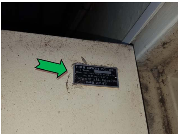
Photo 5. Exterior, main switch board, fire door – non asbestos-containing door core.
