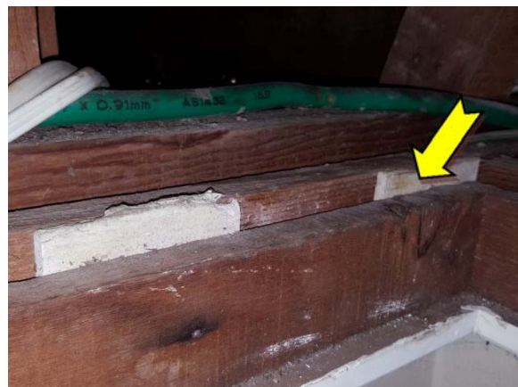
Photo 6. Interior, toilets, packers above ceiling void – non asbestos-containing fibre cement sheeting.
