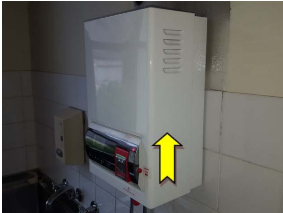
Photo 7. Interior, ground level, kitchen, hot water heater – suspected SMF internal insulation.
