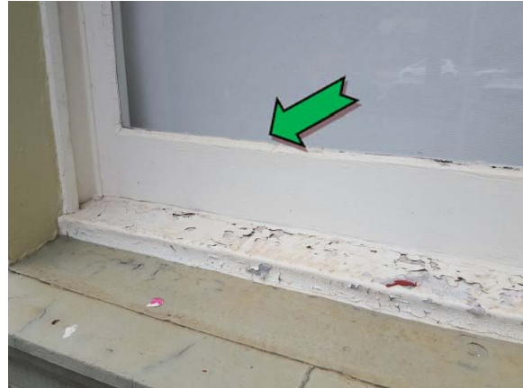
Photo 2. Exterior, throughout, window frames – non asbestos-containing window caulking.
